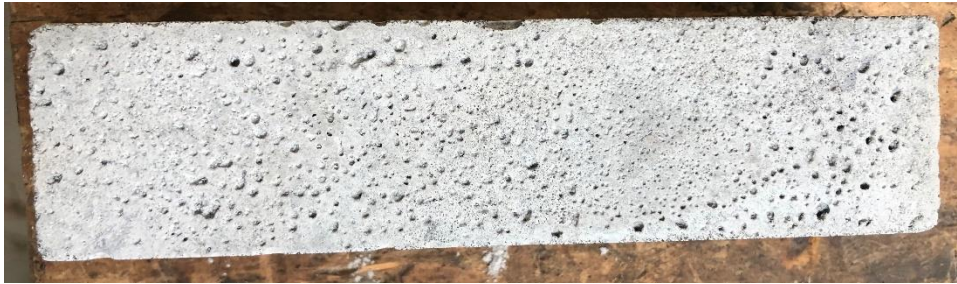
Figure 2.5 Concrete bar with surface treatment.
