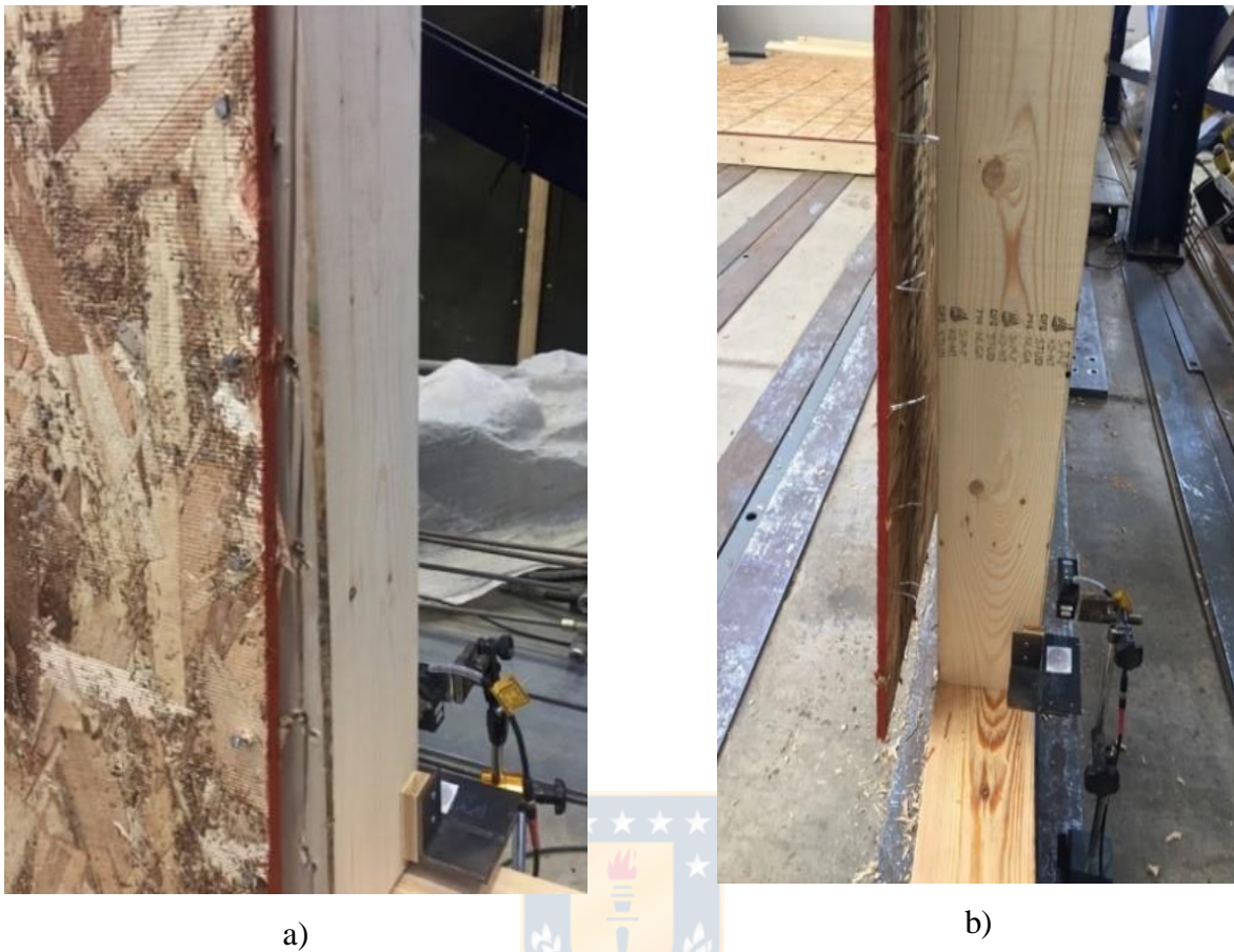
Figure 4.9. Failure modes, nailed (a) and stapled (b) shear walls.
