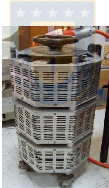
Fig. 4.18. Three-phase autotransformer
