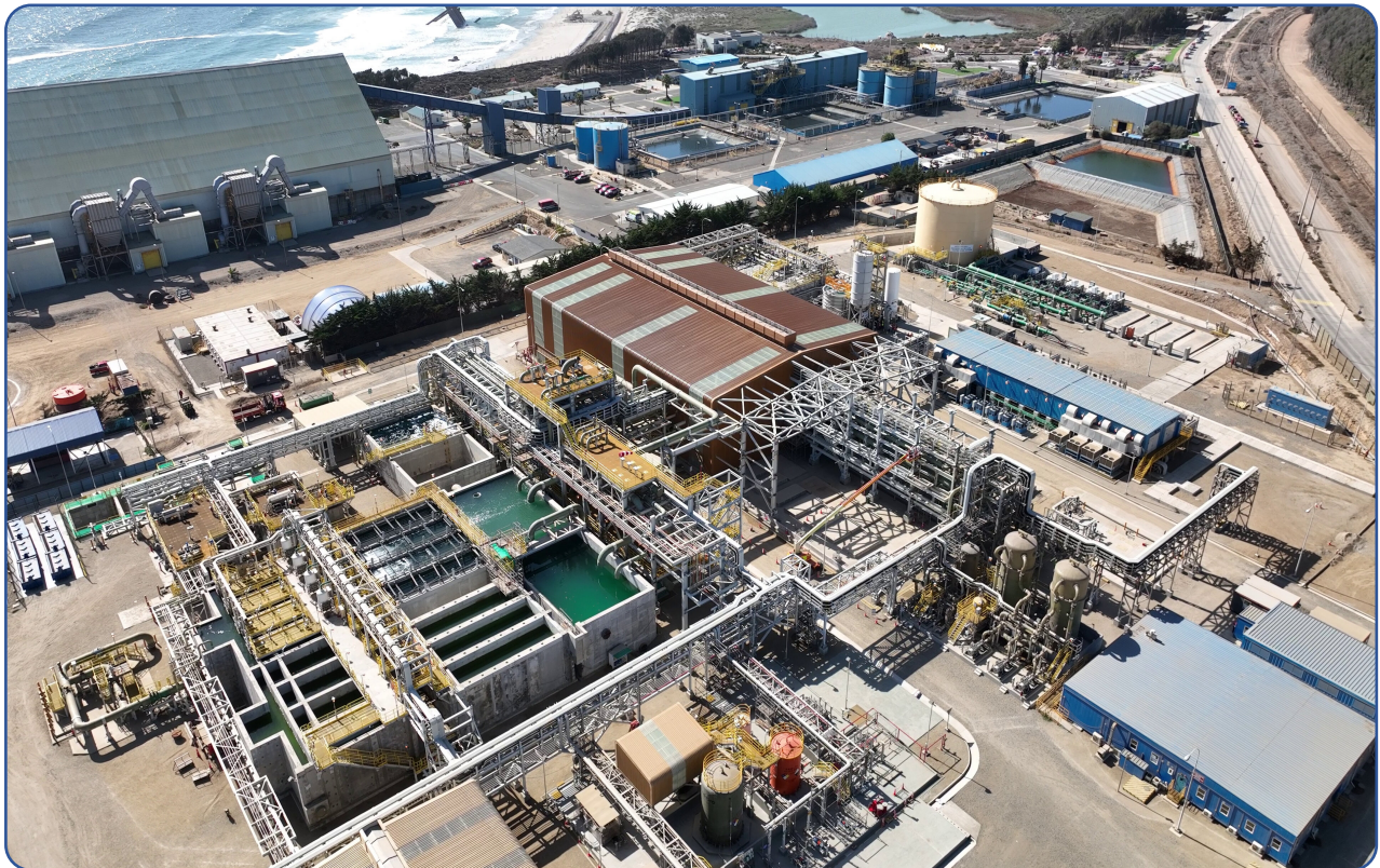
Figure 0-1: Los Pelambres Sea Water Reverse Osmosis desalination plant, Chile. Photograph by Enzo García-Bartolomei.
