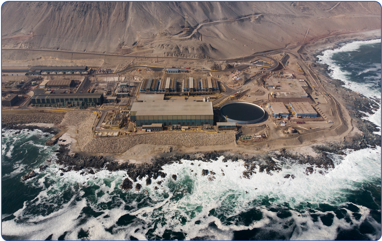
Figure IV-1: Escondida Water Supply 2500 l/s, largest SWRO desalination plant in Latin America. Photograph by Enzo García-Bartolomei.
