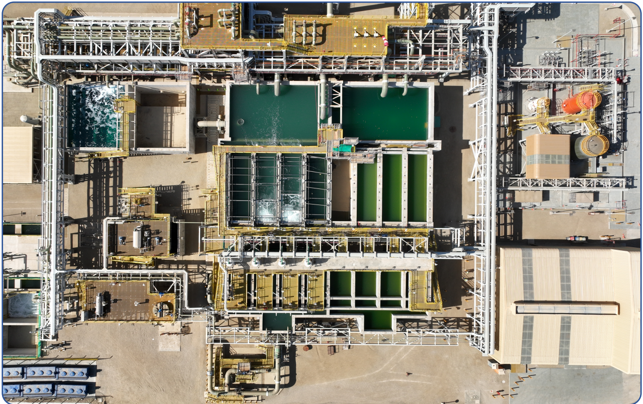
Figure 0-2: Pretreatment system at Los Pelambres Sea Water Reverse Osmosis desalination plant, Chile. Photograph by Enzo García-Bartolomei.
